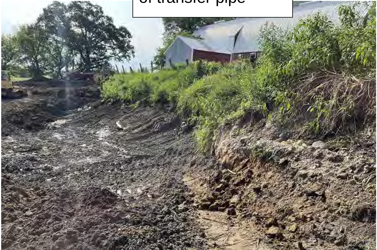
Removal of the end of transfer pipe
